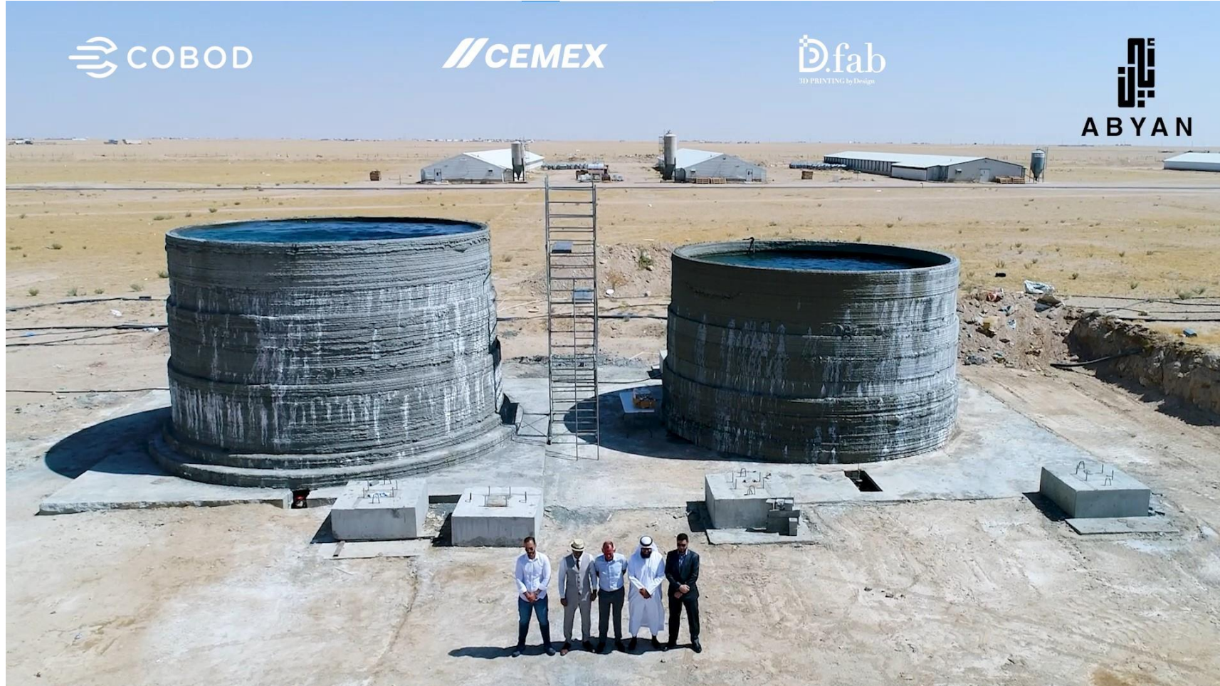
2 chicken drinking water tanks, 4,5m tall and 7m diameter. Kuwait.
