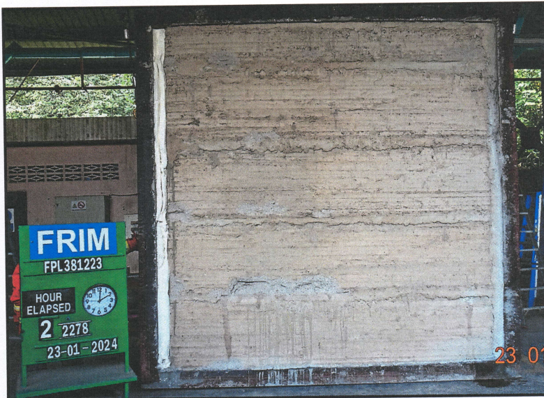
Plate 8. Exposed face after the fire test (Time taken: 120 minutes).
