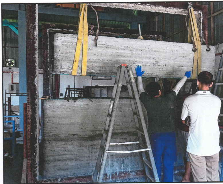
Plate 1. Construction of the 3D Printed Wall.
