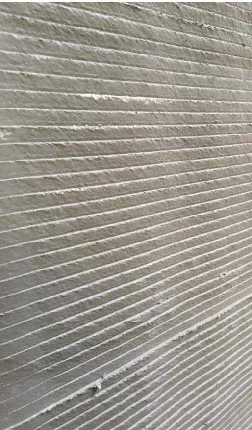
Mortar – 1 inch (2.5 cm) layer
