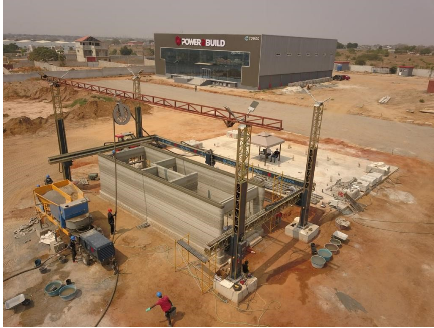
Fig. 6. Power2Build's site in Luanda, Angola and home to the first building 3D printed with the D.fab concrete solution. The printer – in the middle – and the batch plant – to the left – has been set up to print the building.
