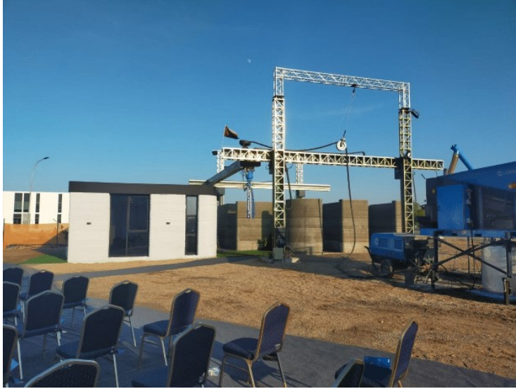
Fig. 12. A COBOD printer set up in Muscat, Oman around the second part of the social housing building after having completed the first part.
