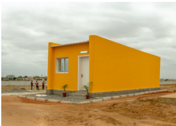
Fig. 8. The finished 53 m2 house in Luanda, Angola. The first 3D printed building with the D.fab concrete solution.
