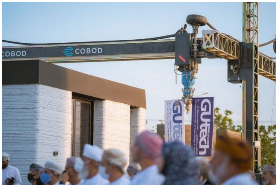
Fig. 14. Inauguration of the building in Muscat, Oman. The third and with the 195 m 2 , the largest 3D printed building made with the D.fab concrete solution so far.
