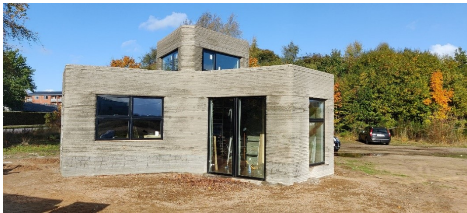
Fig. 11. The printed 37 m 2 tiny house in Holstebro, Denmark. The second 3D printed building with the D.fab concrete solution.
