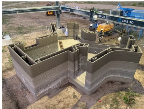
Fig. 9. The printer set up in Holstebro, Denmark to print the second 3D printed building with the D.fab concrete solution.
